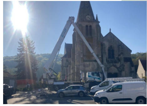
installation de la protection anti-pigeon
